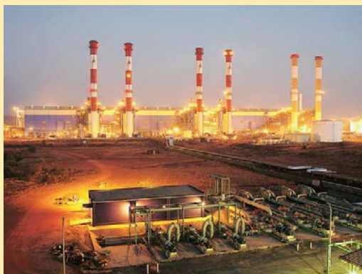
Figure 7.8. The Dabhol Power Plant. Credit: © 2015 by Business Standard
